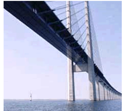
Figure 43: Tolled Øresund bridge in Denmark
