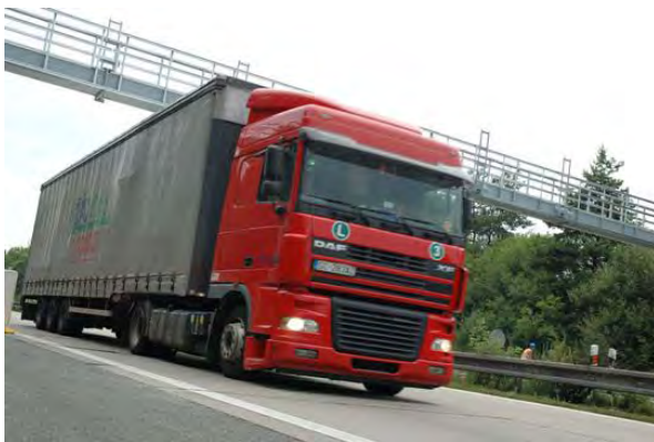
Figure 8: Tolling gantry in Czech Republic
