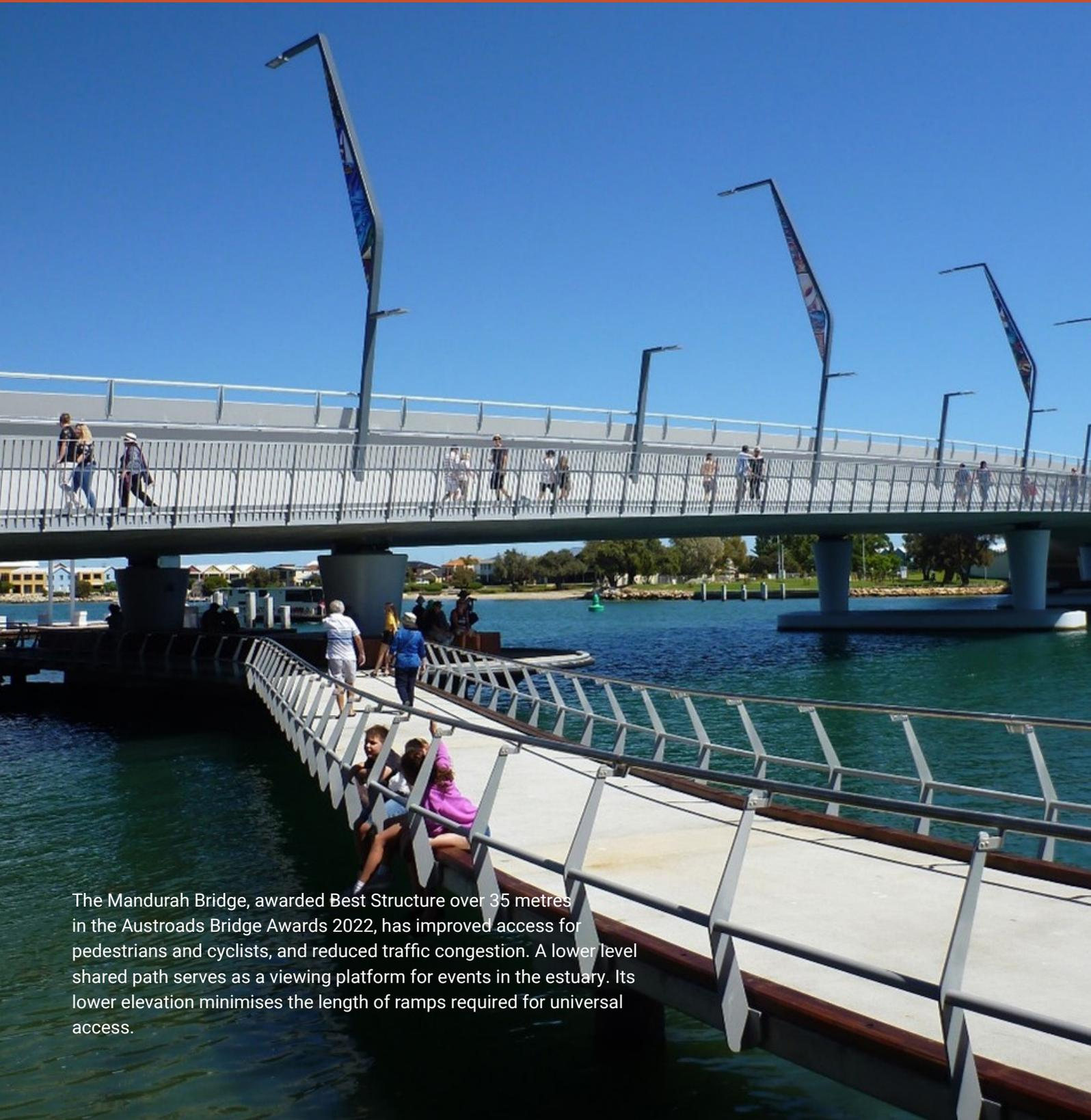
The Mandurah Bridge, awarded Best Structure over 35 metres in the Austroads Bridge Awards 2022, has improved access for pedestrians and cyclists, and reduced traffic congestion. A lower level shared path serves as a viewing platform for events in the estuary. Its lower elevation minimises the length of ramps required for universal access.
